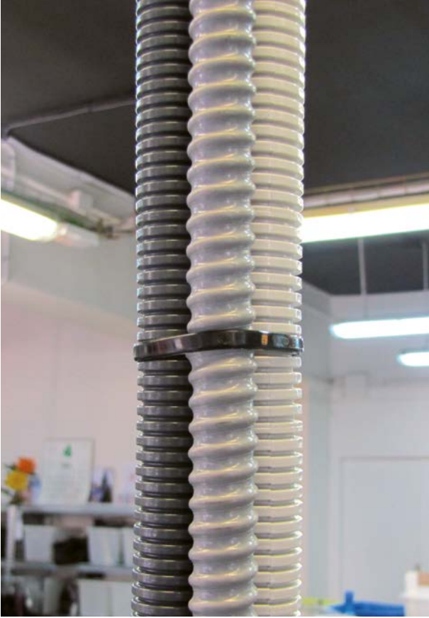
Work spaces: office
