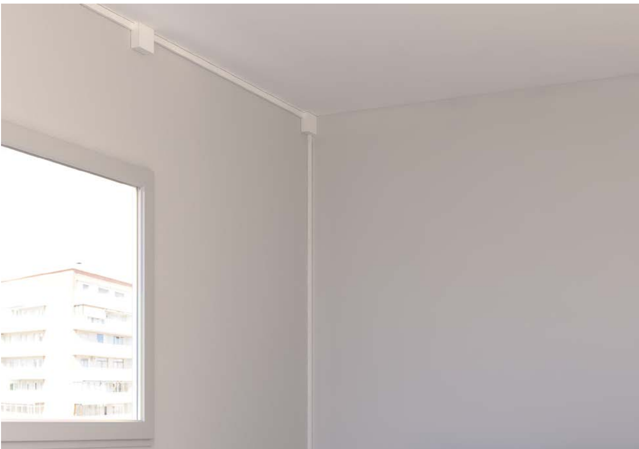
Apartment building renovation
