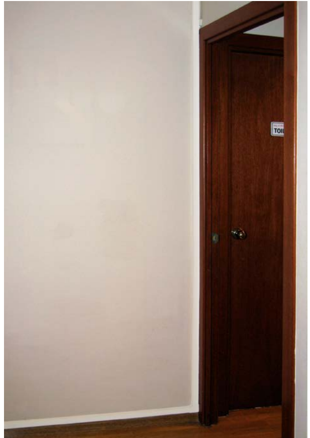
Apartment building renovation
