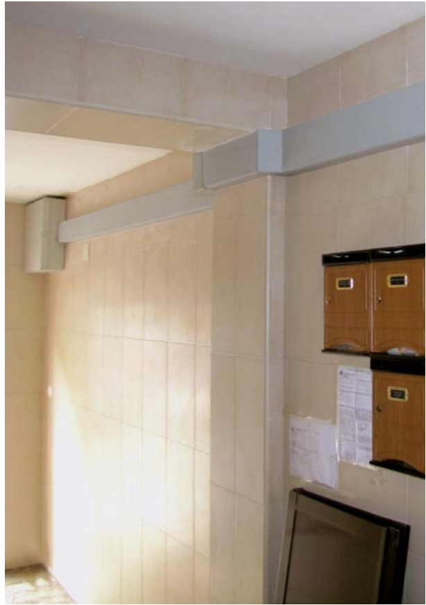
Apartment building renovation
