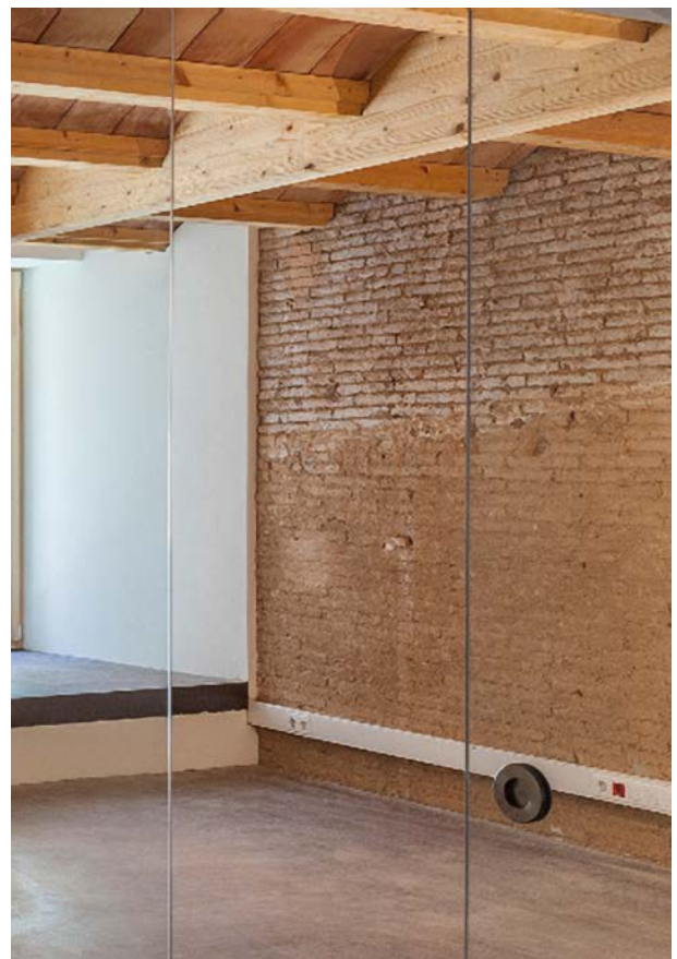
Work spaces: office renovation
