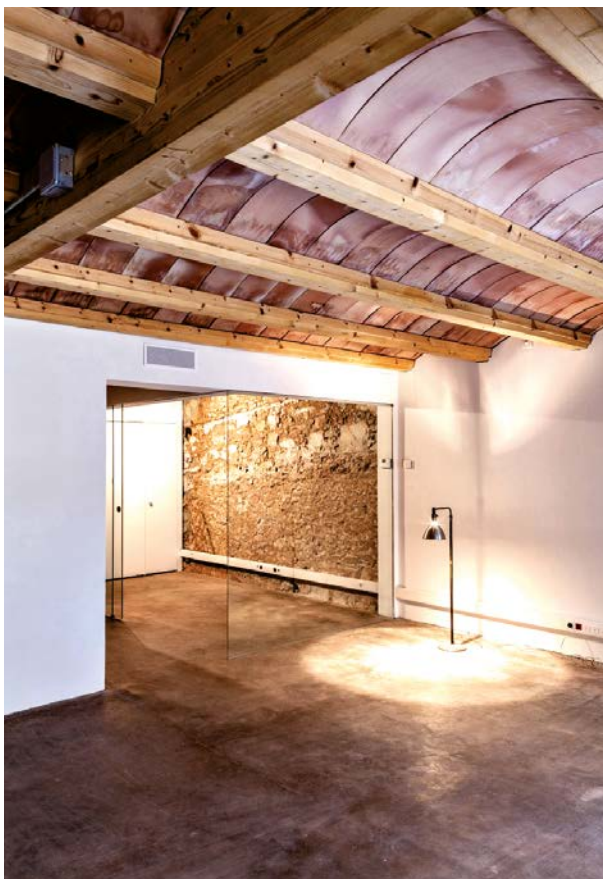
Work spaces: office renovation
