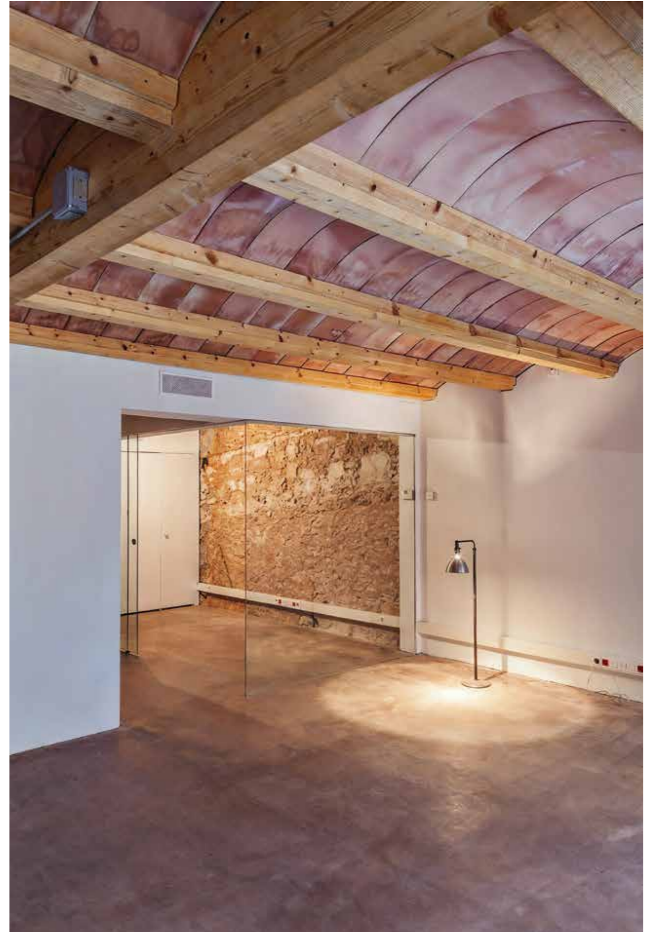
Work spaces: office renovation
