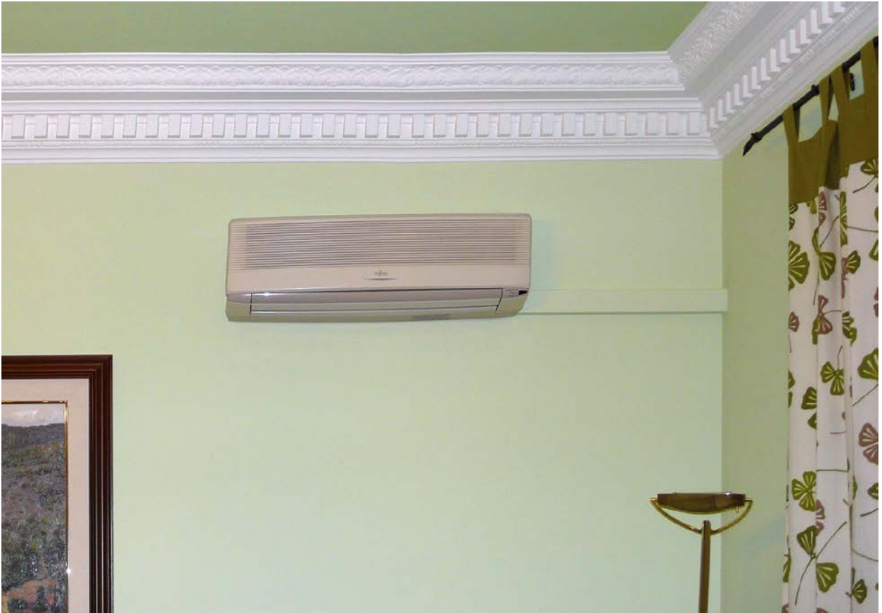
Apartment building renovation
