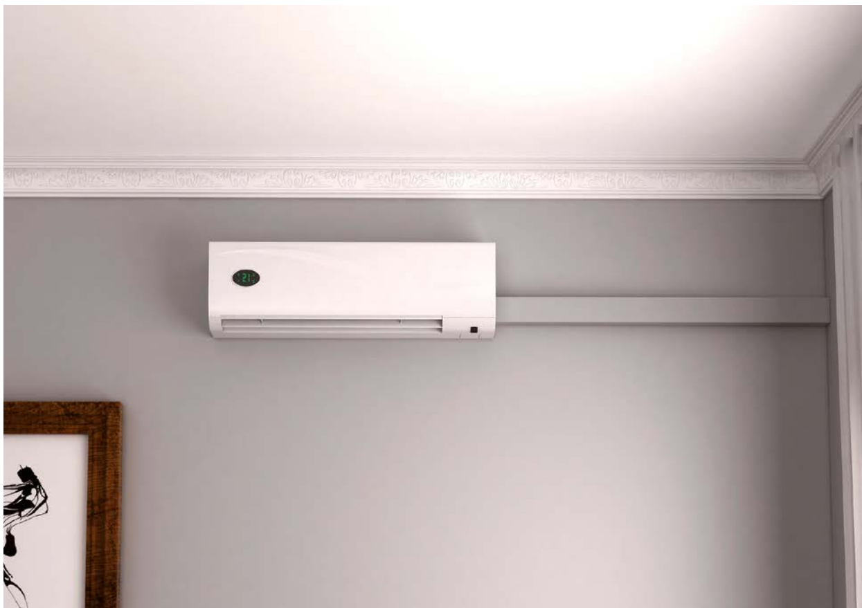
Apartment building renovation
