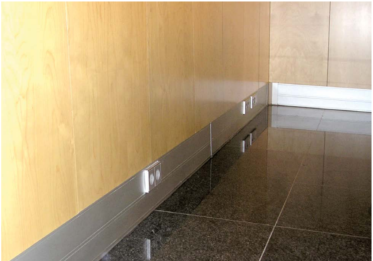
Work spaces: office
