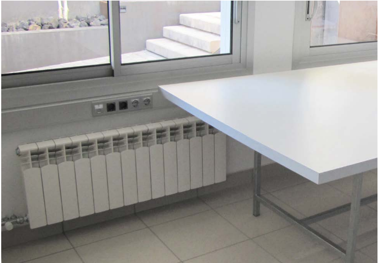
Work spaces: office
