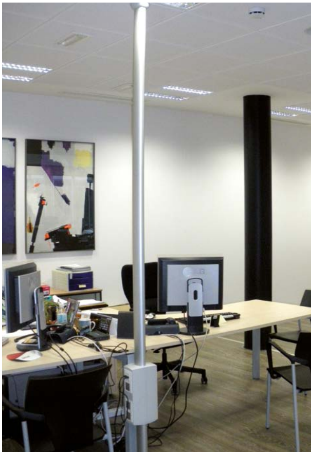
Work spaces: office
