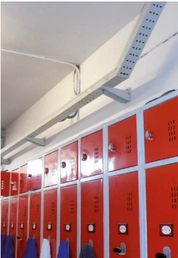
Industrial building: dressing room
