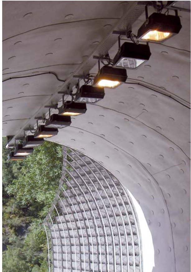
Road infrastructure: tunnel
