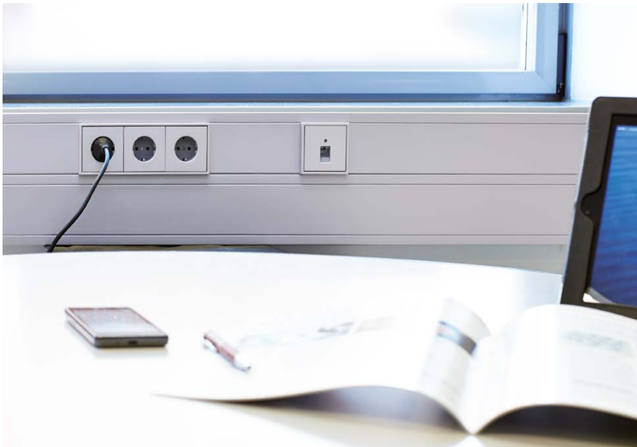
Work spaces: office
