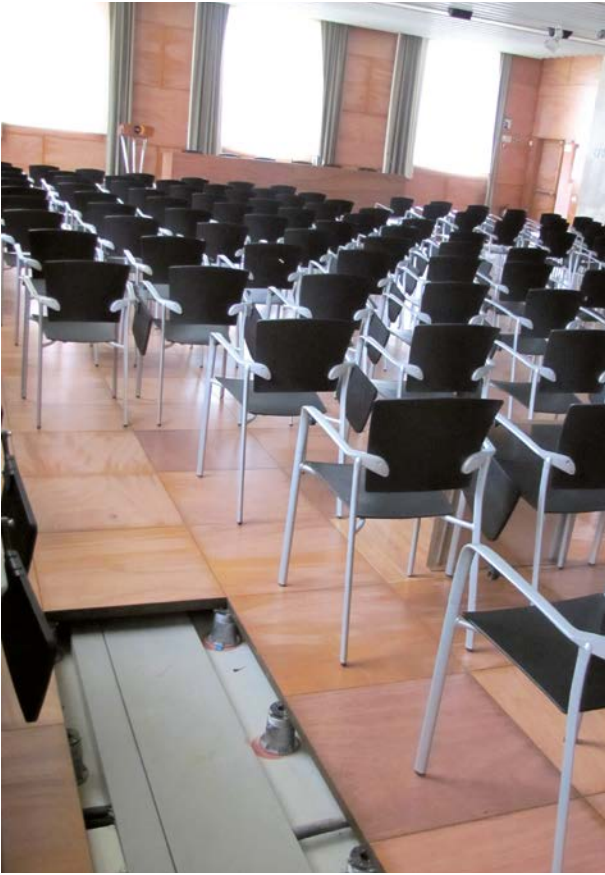
Work spaces: conference hall
