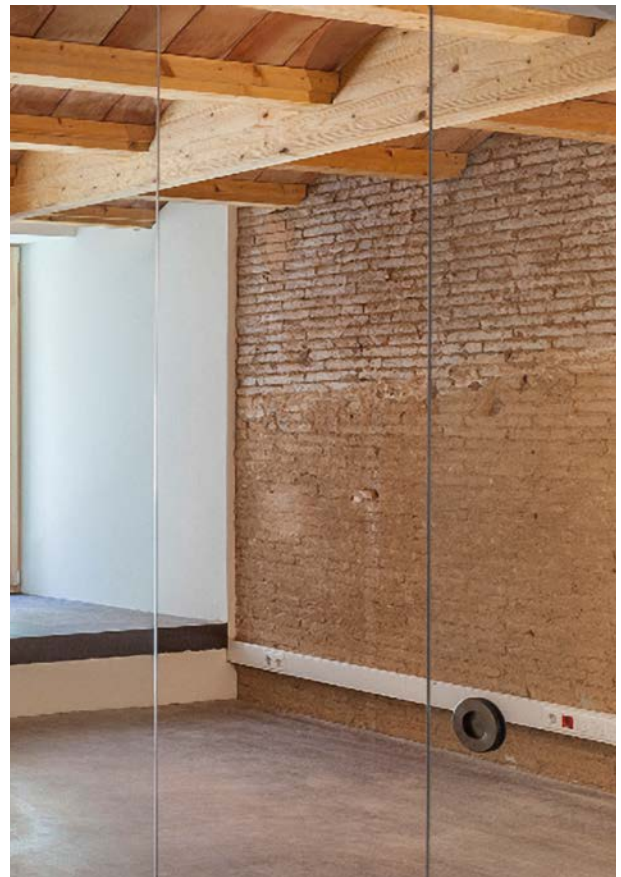
Work spaces: office renovation
