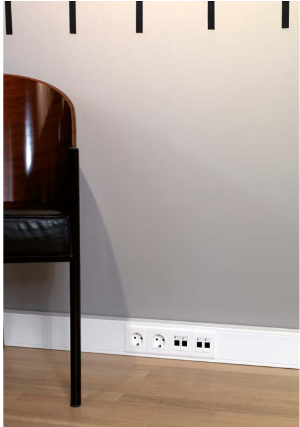
Work spaces: office
